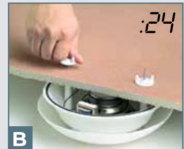
B Two (2) wide-based wing nuts secure the speaker assembly to the ceiling tile.
